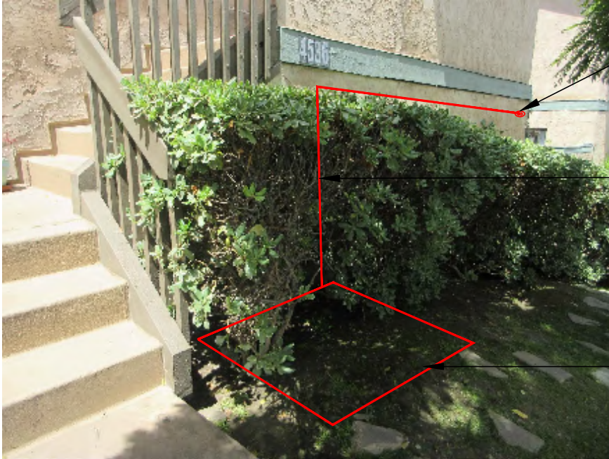
PROPOSED CONDITIONS AT UNIT 4536 (EXTERIOR)
